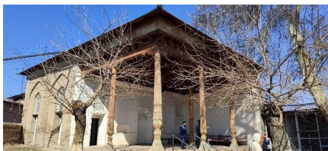
Figure 1. View of the courtyard of the mosque
